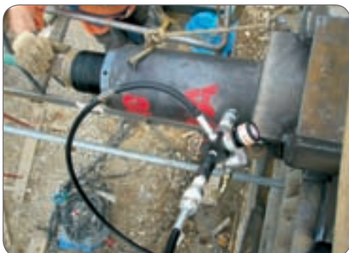
Hollow, single-acting cylinder with safety ring CRM 60/260 GS for bridge launching operations.
