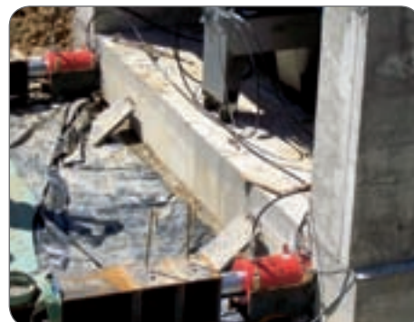
CRIC 250/250 cylinders for shifting a prefabricated concrete structure.
