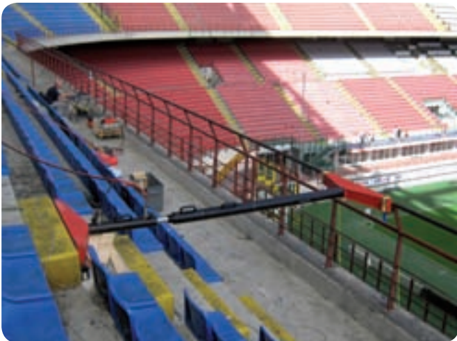
Equipment for lateral stress tests for safety components during the stages, by means of an F.P.T. kit made of aluminium cylinders, extensions, cross supports and hydraulic pump.
