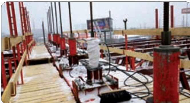
Lifting sections of concrete structure bridges using 60 ton-capacity hollow cylinders and traction bars.
