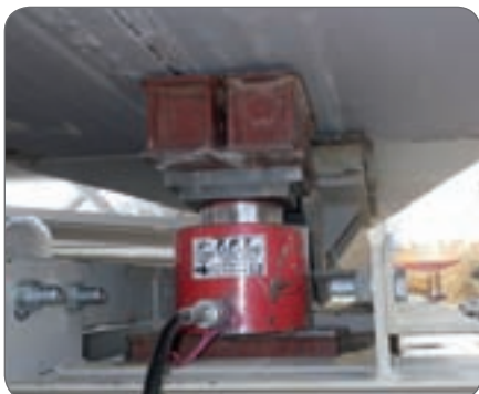
100 ton-capacity compact cylinder - Model F.P.T. CRM100/50C 100 ton capacity, 50 mm stroke
